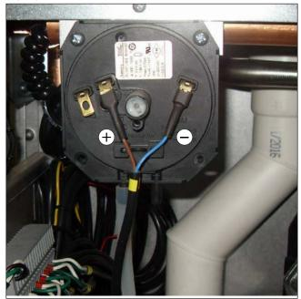
Fig. 20 Flue pressure switch
