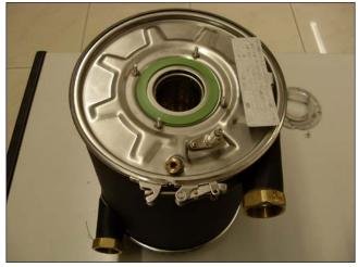
Fig. 5 Heat exchanger (fan motor removed - note location of green burner gasket)
