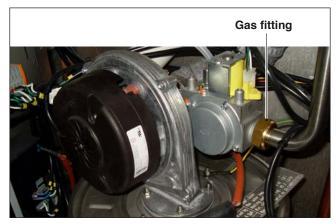
Fig. 48 Gas fitting - model SSB85 - SSB120
