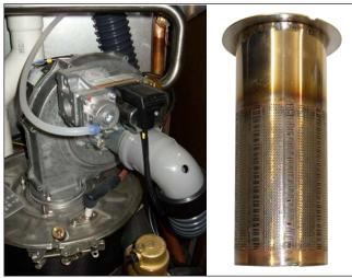
Fig. 4 Burner head
