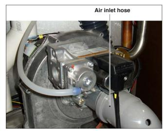
Fig. 64 Air inlet hose SSB160
