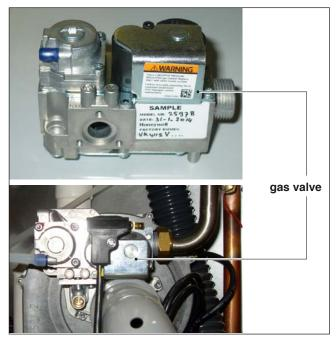
Fig. 16 Gas valve SSB160
