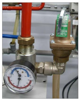
Fig. 22 Pressure relief valve (pipe connection from boiler supply to relief valve is field supplied and does not come with the boiler).
