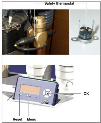
Fig. 12 Manual reset High Limit Safety Thermostat
