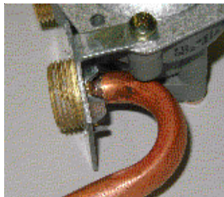
Figure 3 Detail of hot water outlet pipe and bracket (step C4)
