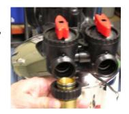
Place the bypass valve is the "Service" or "Bypass" position to test solder joints.
